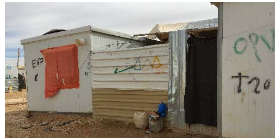
Fig. 7 A covered window to protect the privacy [13]
