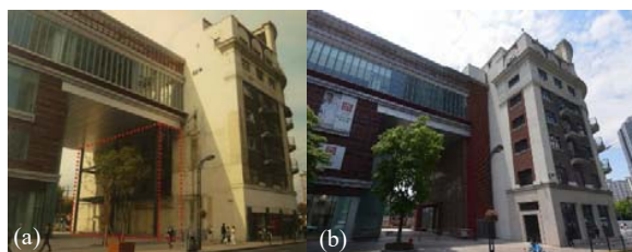
Fig. 6 (a) Photo of the south façade of Hongkou Building before renovation taken on 2012, (b) after renovation taken on 2016
