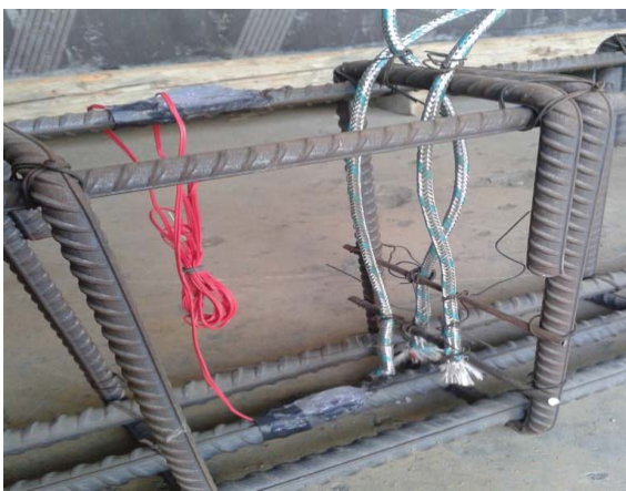
Fig. 2 Location of thermocouples at beams midspan
