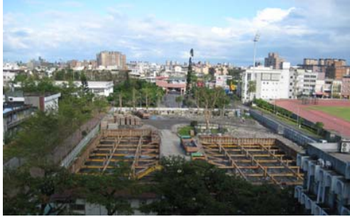
Fig. 2 Excavation construction support
