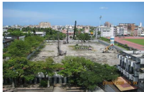
Fig. 1 Excavation construction site
