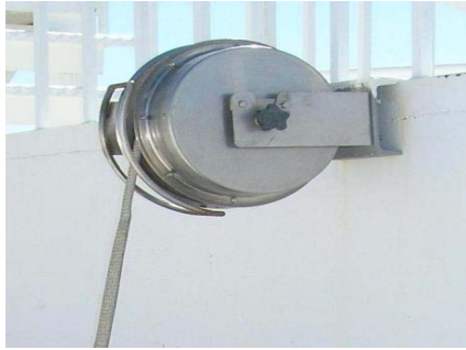
Fig. 3 LEC Retractable Grounding Assembly (RGA) on Floating Roof Tank [1]
