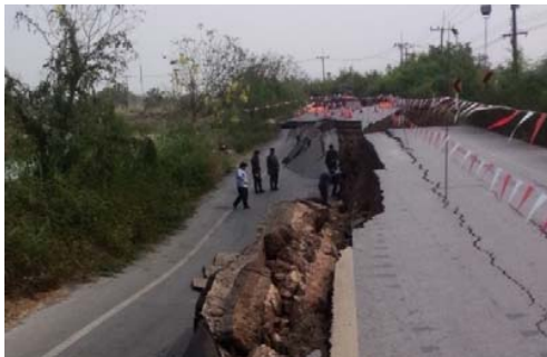
Fig. 1 Road along the canal no.13 collapsed
