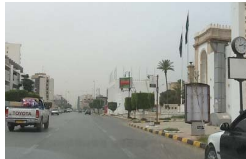
Fig. 3 Roads and sidewalks are in bad condition in OMS [5]
