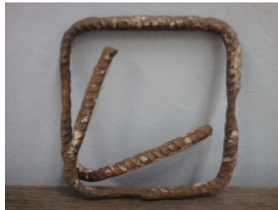
Fig. 7 Typical corroded column stirrup
