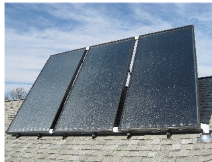
Fig. 1 Flat Plate Collector
