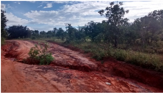
Fig. 8 Access road to the city of Mateiros
