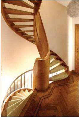
Fig. 8 Corkscrew stairs with a parapet in limba panels and Oak fishbone parquet with wengé boarder
