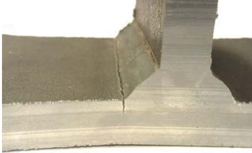
Fig. 2 Crack at weld toe [1]
