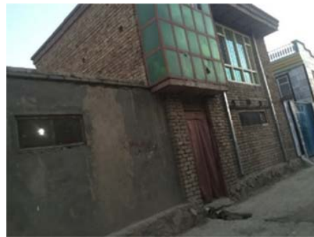
Fig. 12 Sample of masonry building
