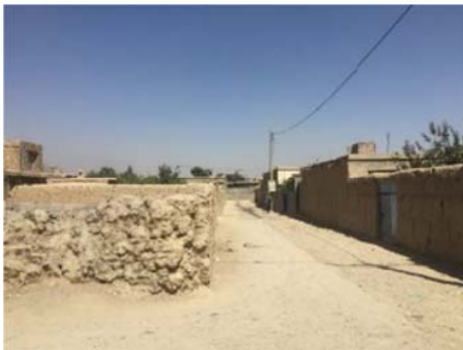
Fig. 11 Sample of an adobe building
