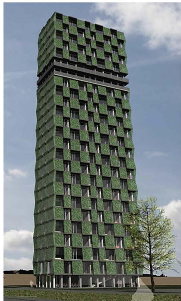
Fig. 7 Proposal for new cladding with solar ivy, south and west elevation [9]
