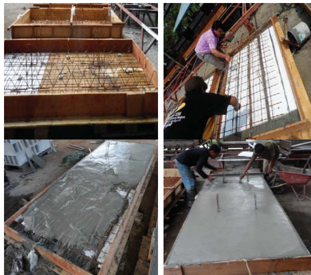
Fig. 3 Preparation, fabrication, and casting of PFCSP specimens
