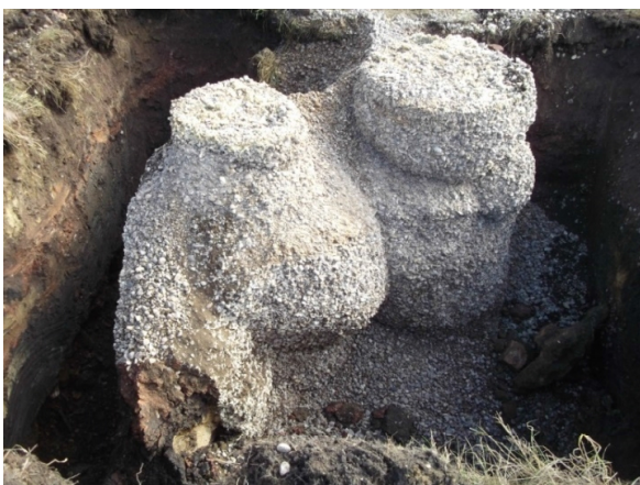
Fig. 1 Photograph of excavated TP02 showing polyurethane resin foam migration through 10 mm pea gravel fill
