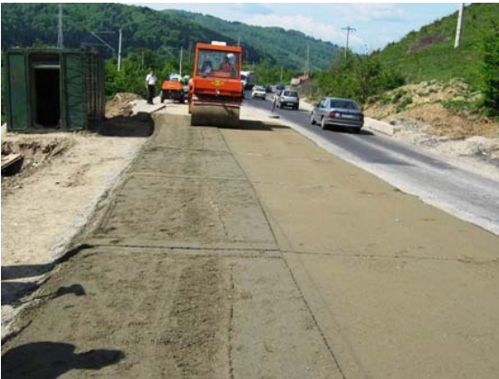
Fig. 1 Roller compacting
