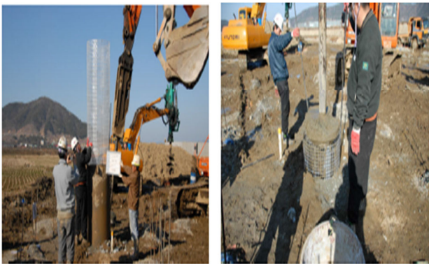
Fig. 6 Construction GESC at the site
