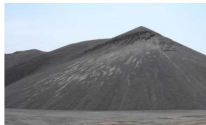
Fig. 2 Stockpiling of steel slag aggregates at crushing plant
