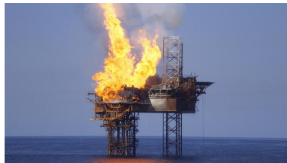
Fig. 2 A major platform fire [17]
