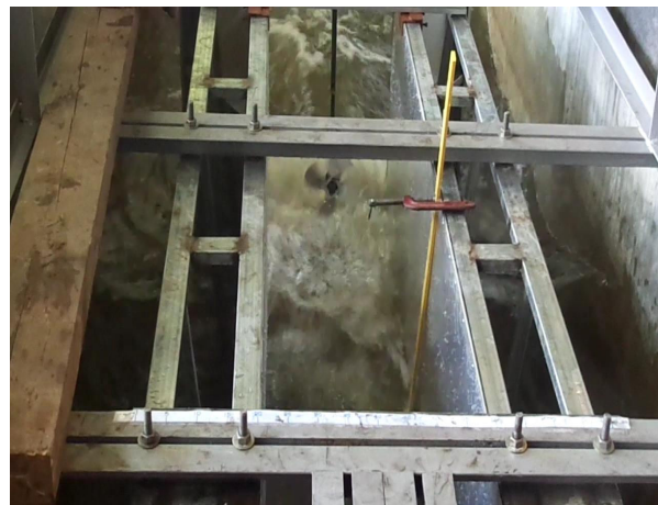
Fig. 6 Turbine placed at the tunnel end
