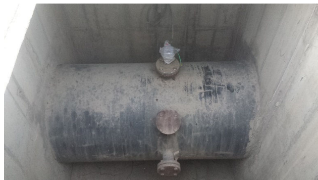
Fig. 8 Mounting position of sensor
