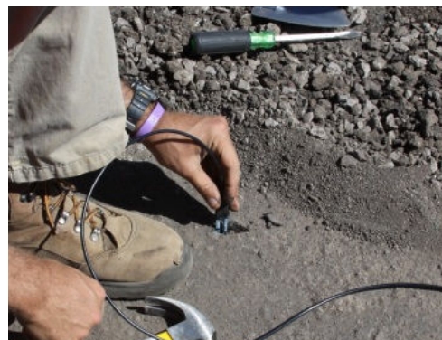
Fig. 3 Installation of a moisture probe
