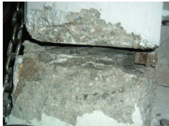
Fig. 1 Cracking of the corbel of the AP1R test specimen
