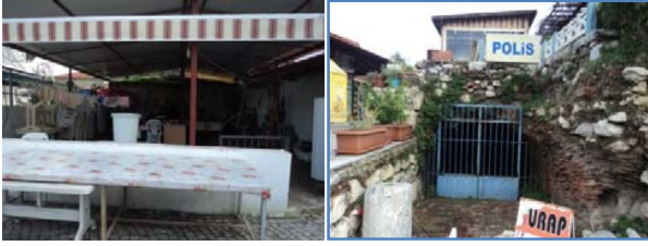
Fig. 6 Important historical buildings in bad condition
