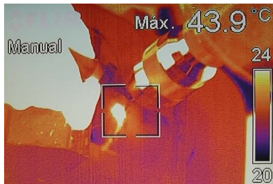
Fig. 9 Example of a thermography image with lubrication collected at the maximum temperature
