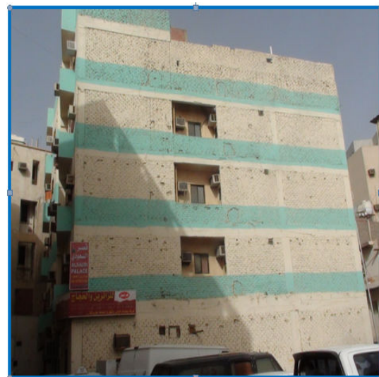
Fig. 3 Side view of the case study building in Madinah
