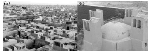
Fig. 5 (a) High density of construction in hot and arid region of Iran, (b) The two-sided wind-catcher and domed roof as reservoir
