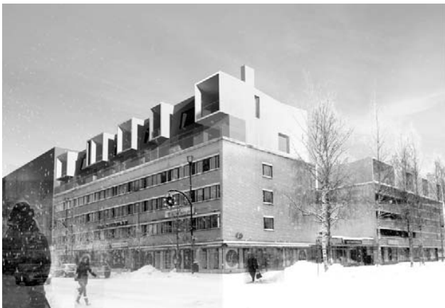
Fig. 12 Additional stories on top of existing buildings, Kirkkokatu 18
