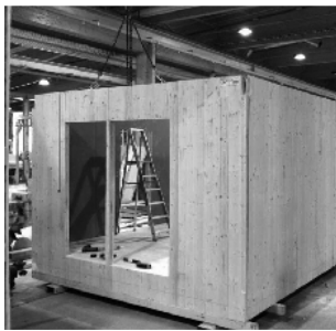
Fig. 6 Fabrication of CLT module elements
