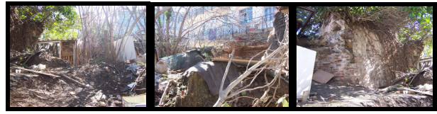
Fig. 11 The bath's interior filled with soil and garbage, the upper parts of the bath walls completed with random stones and the trees blooming out of these - 2014
