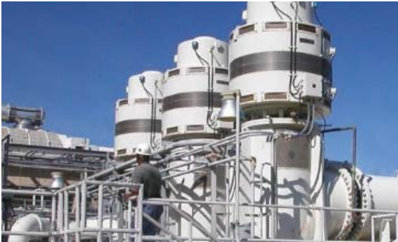
Fig. 1 Typical sea water vertical Centrifugal lift Pumps
