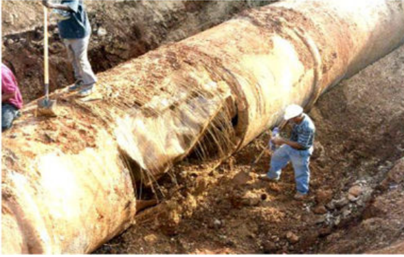
Fig. 2 Transient-caused failure, Super-aqueduct of Puerto Rico
