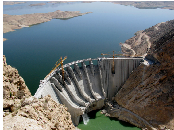
Fig. 3 Salman Farsi (Ghir) dam is a 125 m high concrete gravity arch dam within the Ghareh Agahaj River (northeast view)
