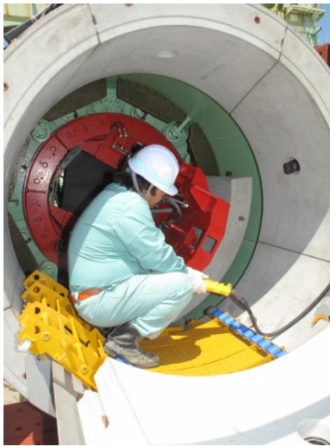
Fig. 6 Secondary lining applied RC segment – assembly
