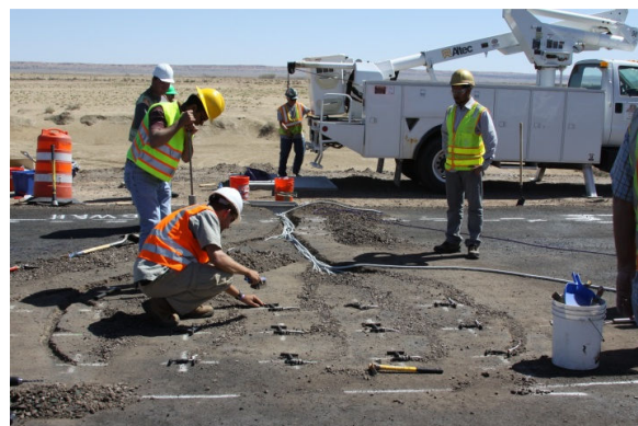
Fig. 3 Installation of horizontal strain gauges
