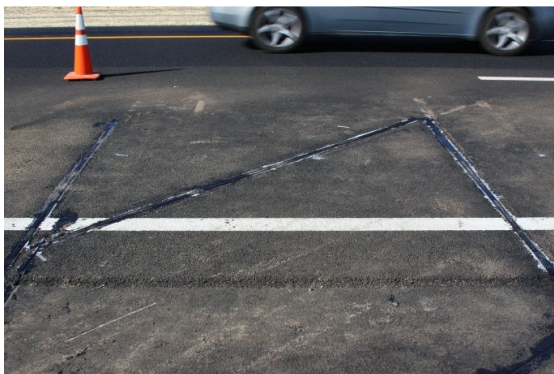
Fig. 5 Installation of axle sensing strips
