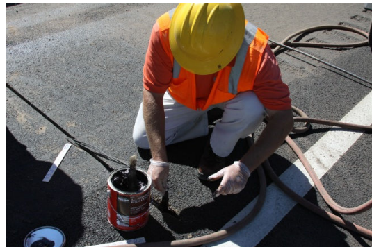
Fig. 6 Installation of temperature probes
