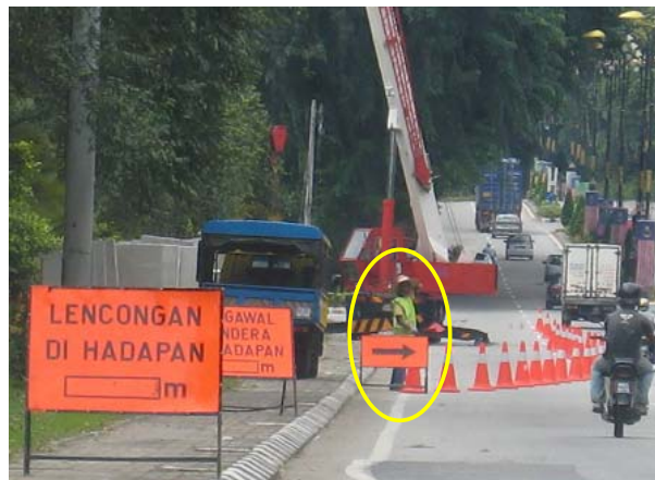
Fig. 1 Flagman is positioned in the work zone
