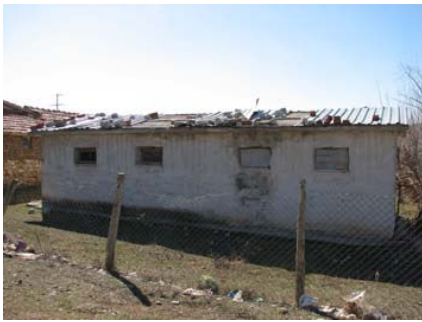
Fig. 4 Cattle shed with it's moved up roof cladding (Kızıllı Village)
