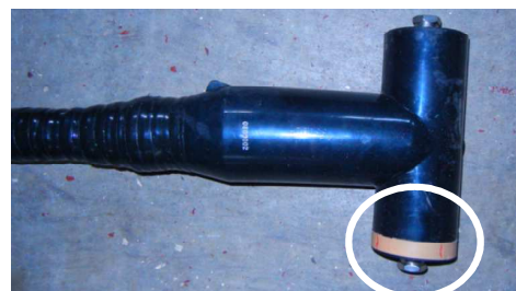
Fig. 3 T-branch joint for a 22 kV distribution system
