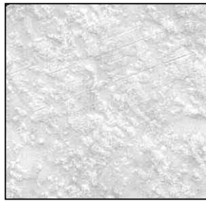
FIGURE 6 THE ORIGINAL IMAGE FOR THE CRACK DEFECT
