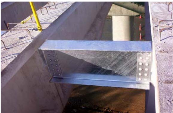
Fig. 3 Steel Cross Beam
