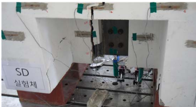
Fig. 8 Crack in SD Type
