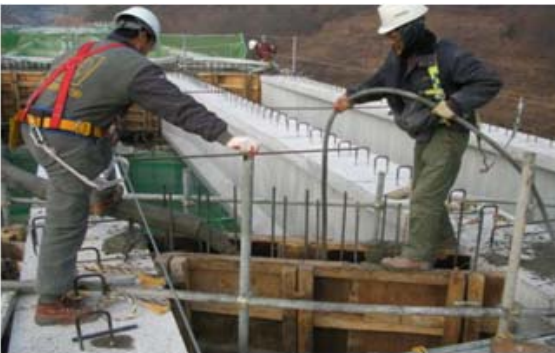
Fig. 2 Placing Diaphragm in Field
