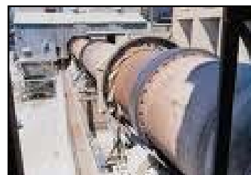
Fig. 1 Rotary Cement kiln
