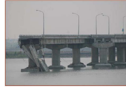
Fig. 18 Case 2: the bridge failure in flood
