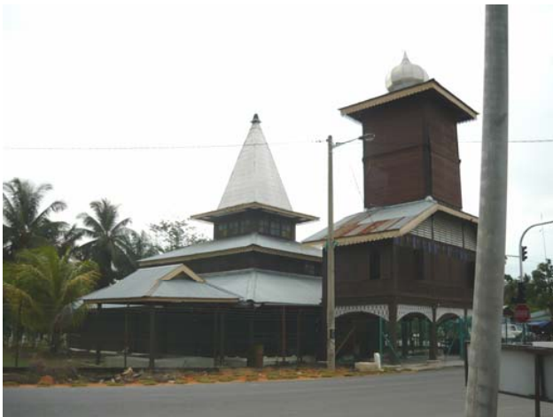
Fig. 1 The conservation of Old Tinggi Mosque, in Bagan Serai
