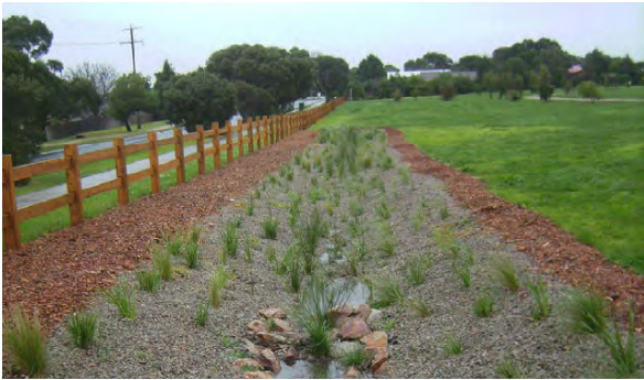
Fig. 2 Bioretention swale Mornington Peninsula Shire Council, Victoria Australia
