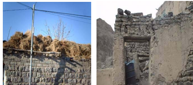
Fig 9 Arranged (left) and unarranged (right) stone wall
