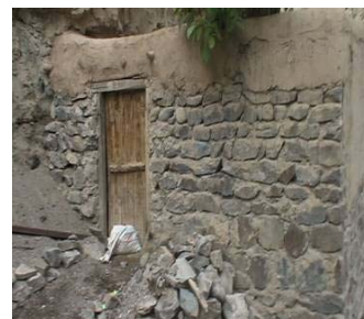
Fig. 6 Stone in the building's walls
