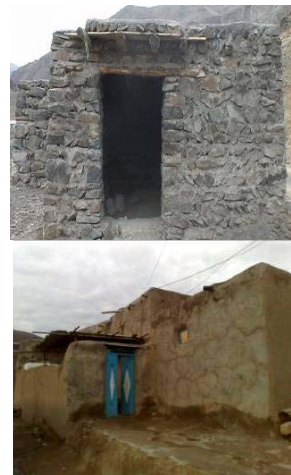
Fig. 1 A house with stone wall (left), A house with adobe wall (right)
