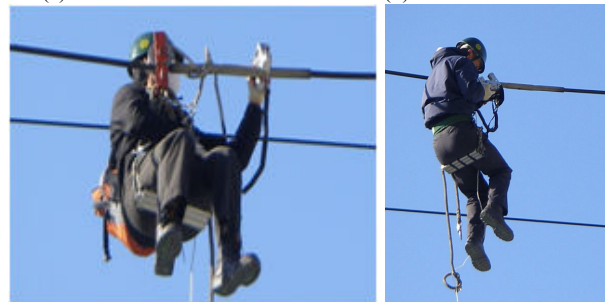
(c) Domestic line sleeve inspect method
