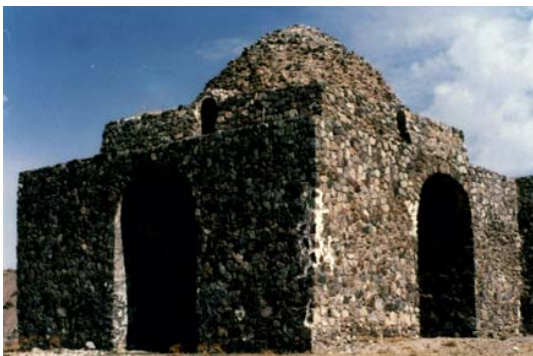
Fig.36 cross-vault "Baze-hur" after mending
