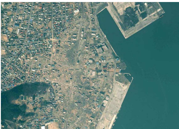
Fig. 3 Aerial photograph of Ofunato city after the Tsunami
