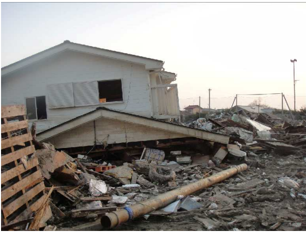
Fig. 8 Failure of the first floor
