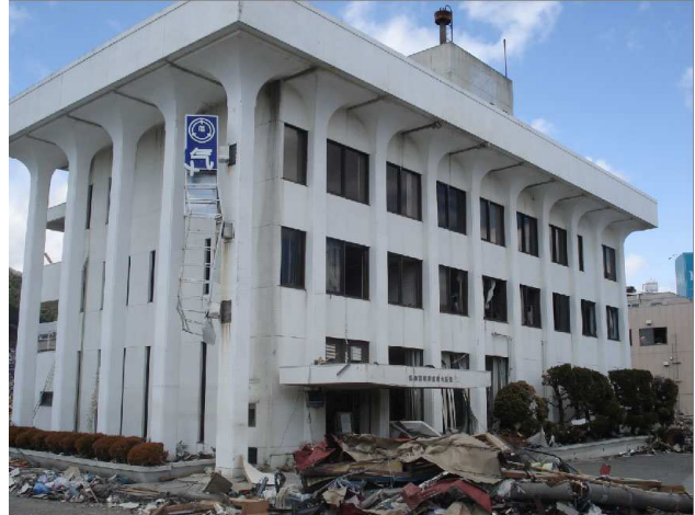
Fig. 15 RC building (Ofunato city)
