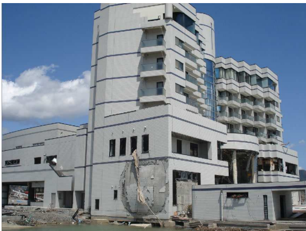
Fig. 19 RC building hotel
