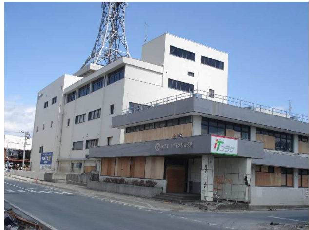
Fig. 16 Two story RC building
