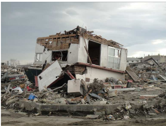
Fig. 10 Over turning of upper floors
