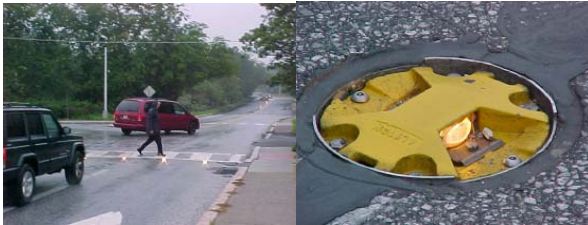
Fig. 9 In-pavement flashing warning lights in Denville [9]
